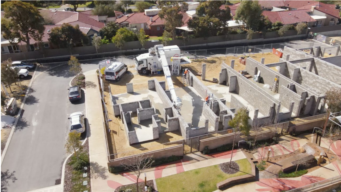
Figure 2.49: Hadrian X ® is a blocklaying machine and system, capable of safely working outdoors in uncontrolled environments with speed and accuracy. Hadrian X ® is pictured here during construction of a 16 two-story townhouse development in Western Australia, the largest construction project ever undertaken by the robot to date. Image credit: FBR Limited.
